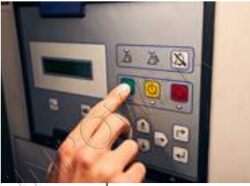
Digital controller with configurable parameters, alarms, and protection
